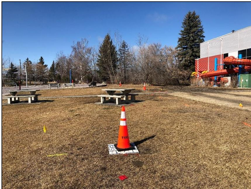
Photo 14: Plywood boards and construction cones placed on top of hydrovaced holes while waiting for survey to arrive.
