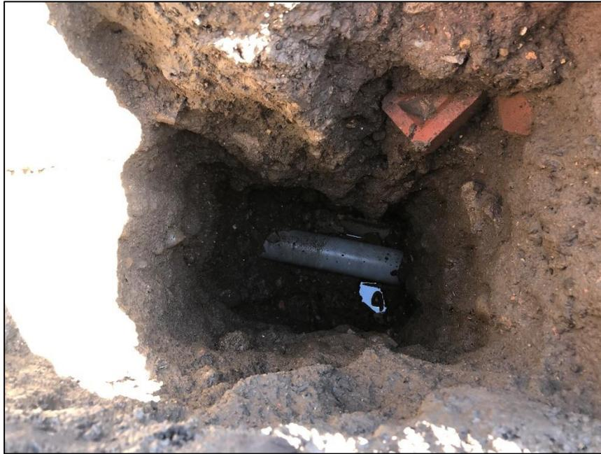
Photo 13: Exposed ATCO utility conduits at location 5. Red clay bricks seen in the excavated hole. Photo taken facing East.
