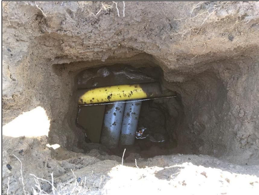
Photo 7: Exposed ATCO and AltaGas utility conduits at location 1. ATCO conduits in grey, AltaGas in yellow. Photo taken facing East.
