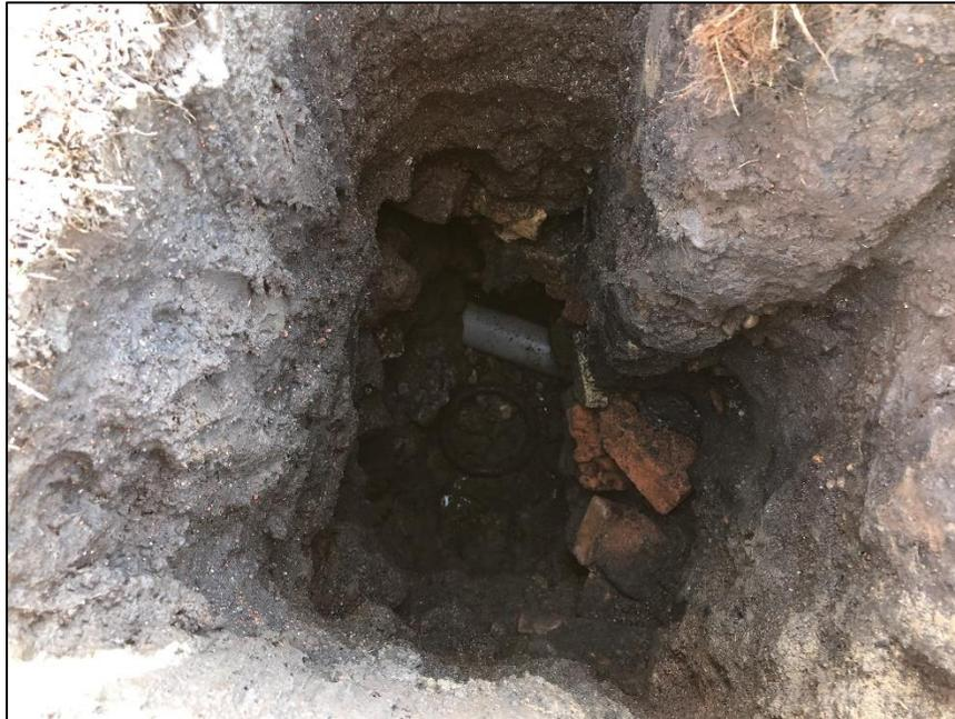
Photo 11: Exposed ATCO utility conduit at location 4. Red clay bricks seen in the excavated hole. Photo taken facing South.
