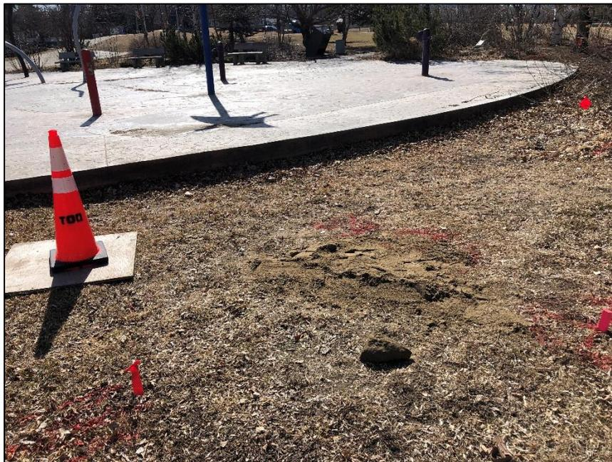
Photo 16: Hydrovaced hole at location 3 backfilled with sand.
