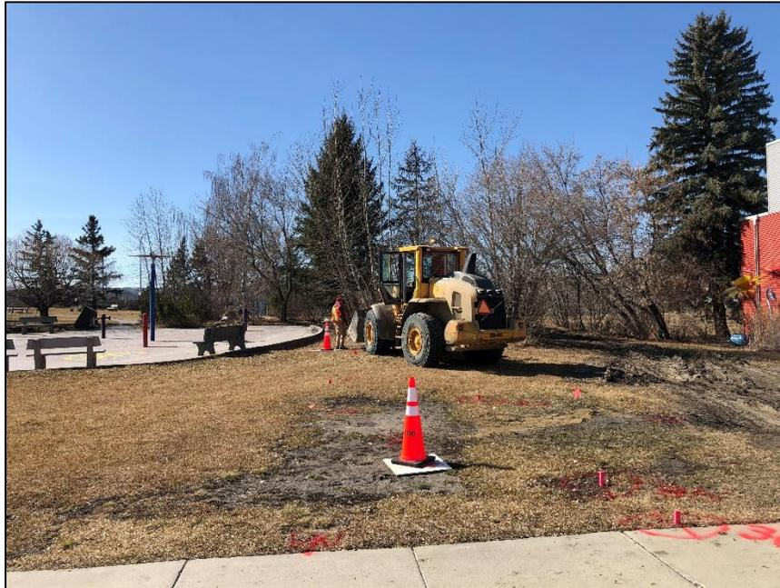
Photo 15: Town of Drumheller backfilling the hydrovaced holes with sand using shovels and a Volvo compact wheeled loader.
