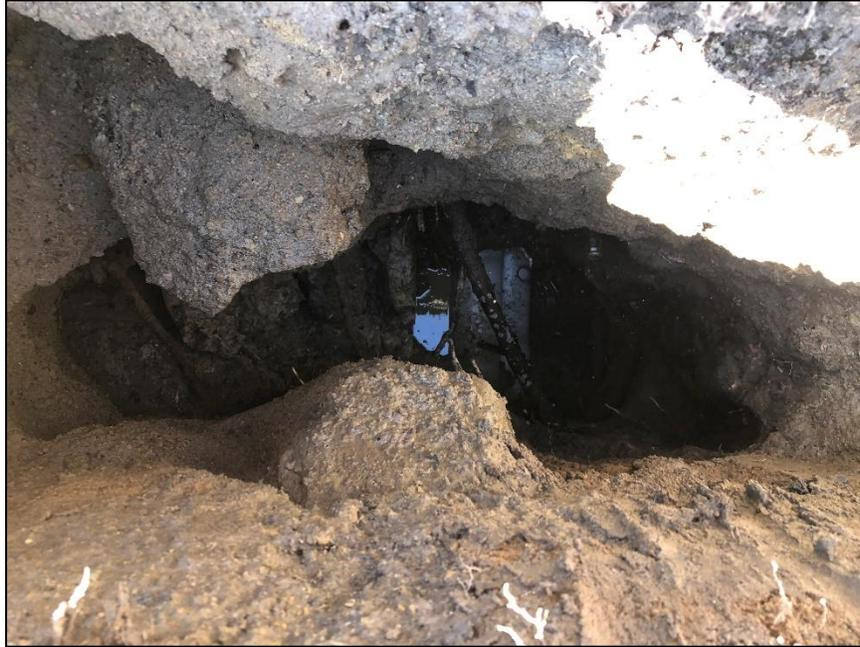
Photo 3: Exposed ATCO utility conduits at location 3. Concrete rubble and abandoned wires above and around the conduit. Photo taken facing East.
