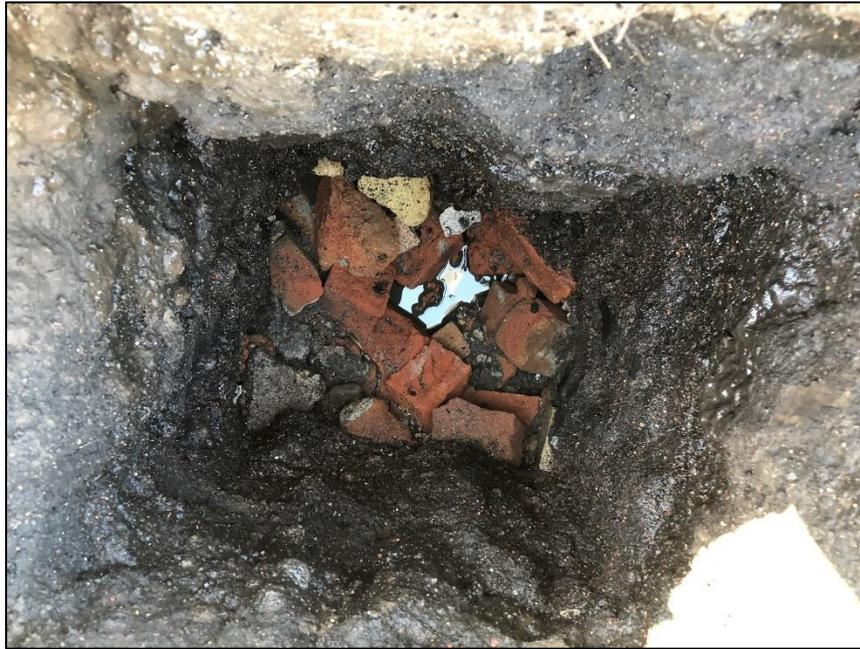
Photo 9: Red clay bricks at approximate depth 0.5 m while hydrovacing at location 4.
