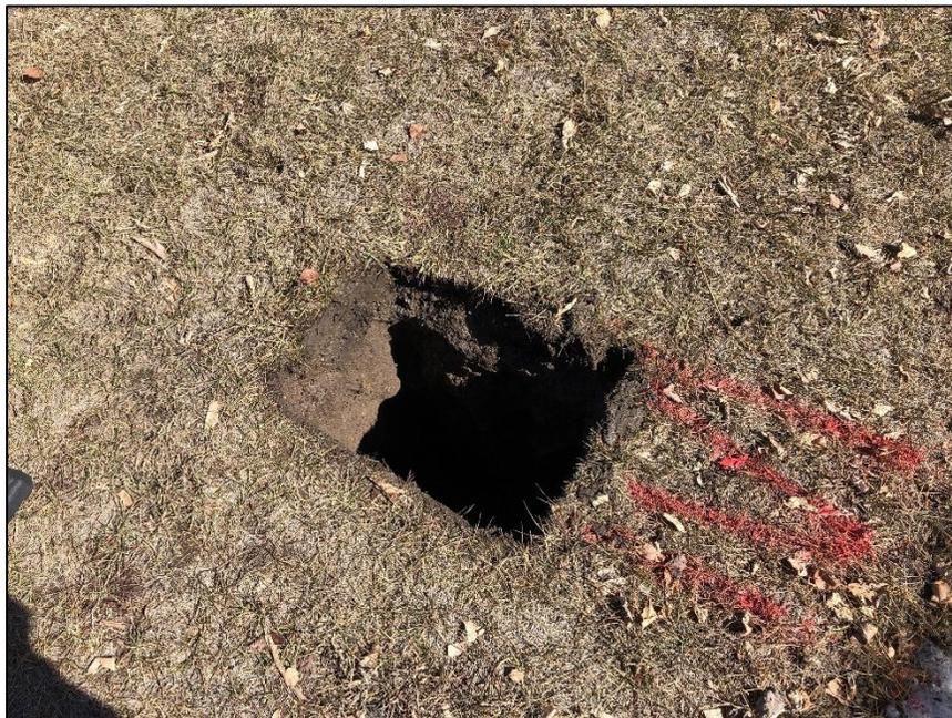
Photo 12: Hydrovaced hole at location 5.
